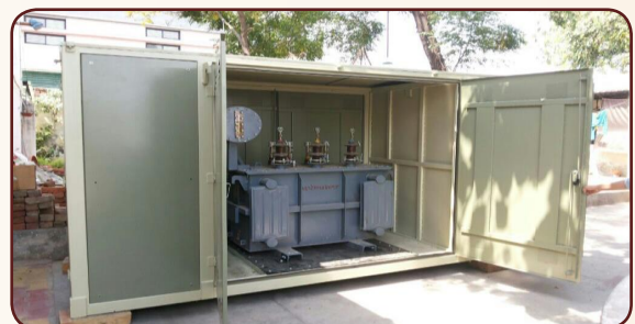
Compact Transformer Cubical
