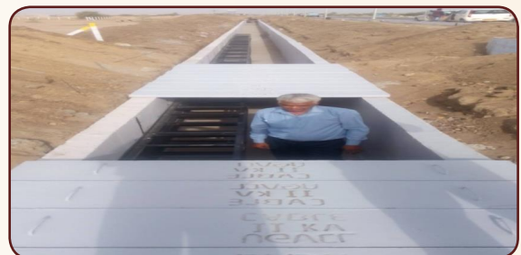
RCC Cable Trench for UG Network
